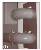
For this type of fitting, it is necessary to ensure sealing around the piping.
